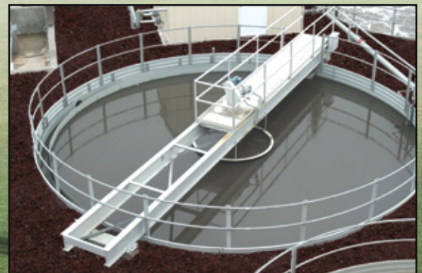
OPTIONAL - MECHANICAL SLUDGE COLLECTOR
