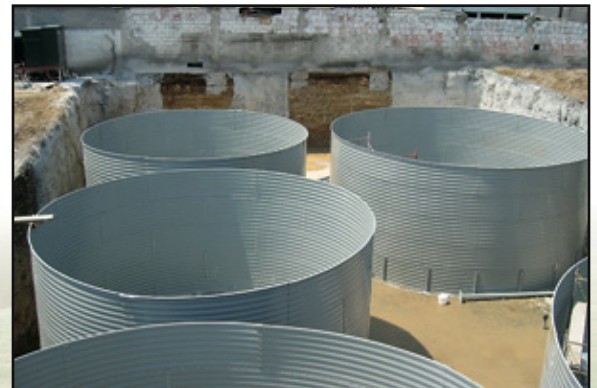
SYSTEM UNDER CONSTRUCTION
