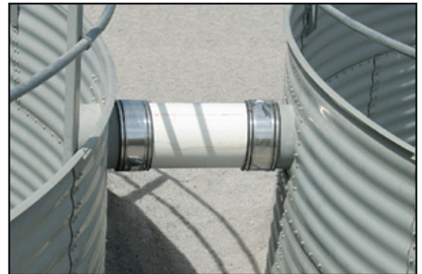
INNER-TANK CONNECTION
